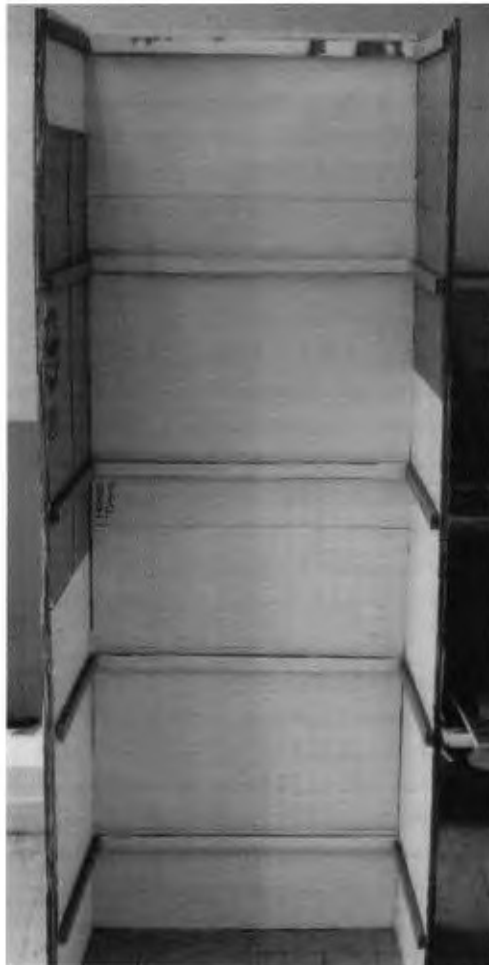
4-43: Back and sides, showing support strips
